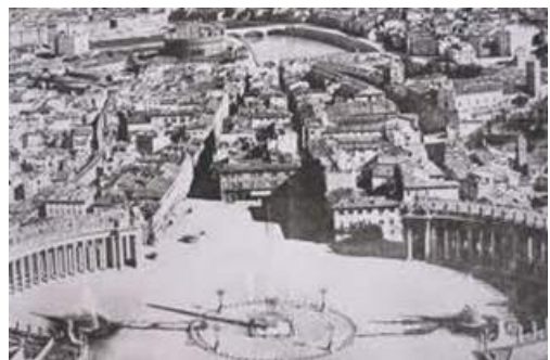
Figure 8. Spina dei Borghi before demolitions (Google images)
