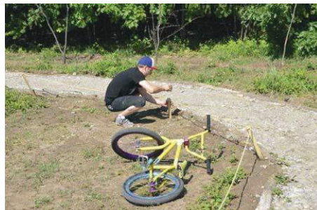
Figure 11. Volunteer helping the construction of pathways
