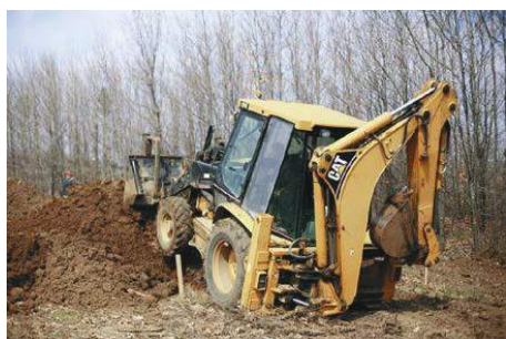
Figure 14. Mechanized execution ramps
