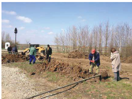
Figure 10. Beginning the work site
